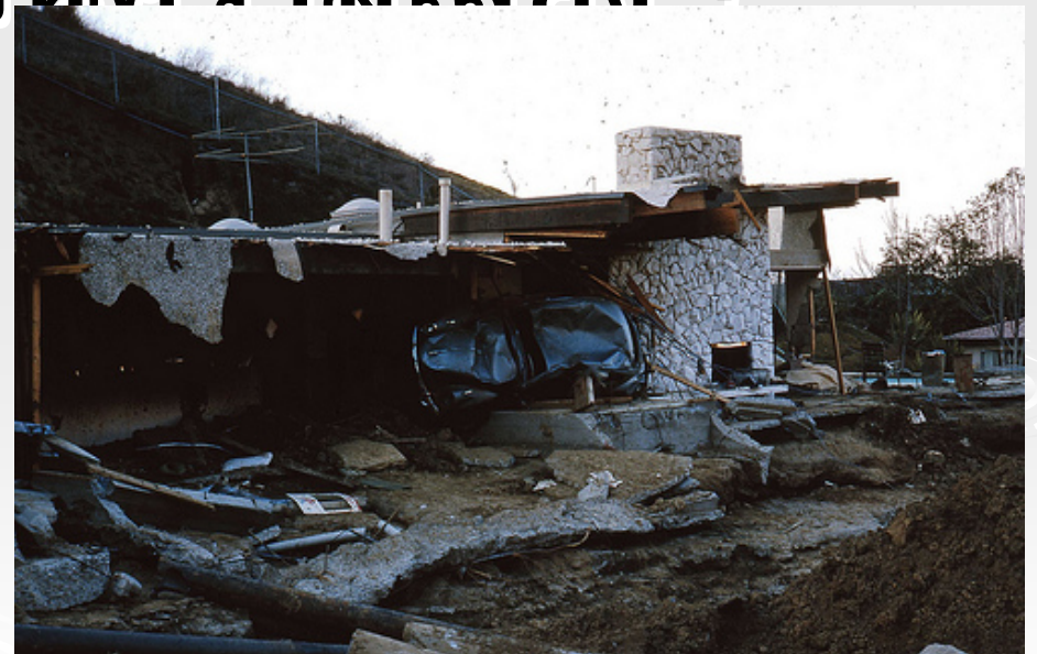
Baldwin Hills Dam failure aftermath
